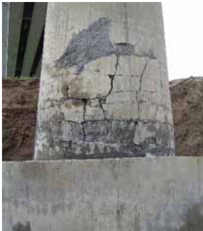
Photo.3 Damage of a pier
