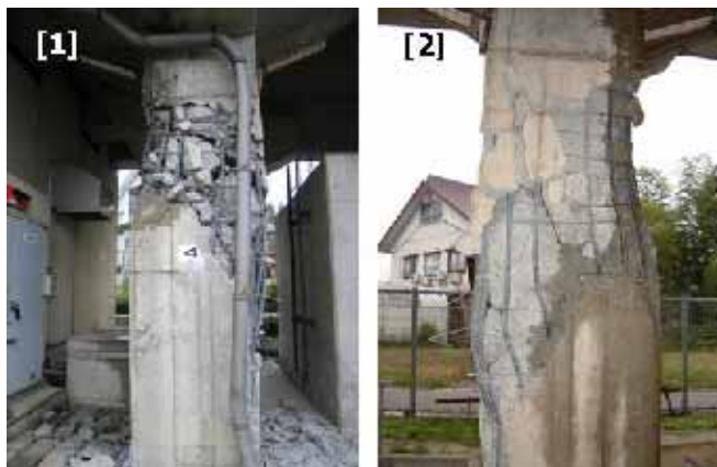
Photo.8 Damage of end column (both sides of a column)
