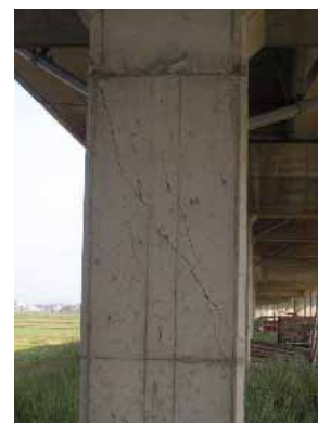
(a) damage of end column (view from a) (b) damage of intermediate column (view from b)
