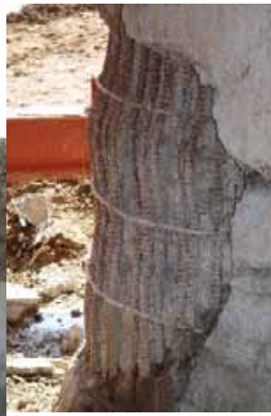
Photo.3 Damage of a pier
