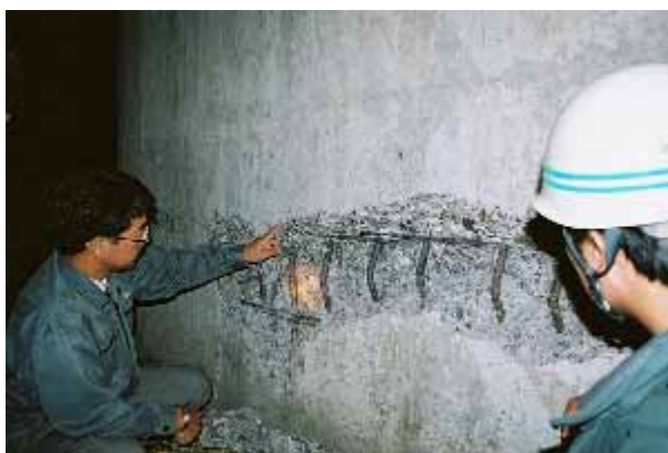
Photo.5 Damage of a pier
