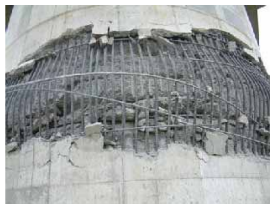
(b) Failure at mid height in pier
