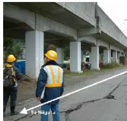
Photo.9 Strengthened column by the steel jacketing
