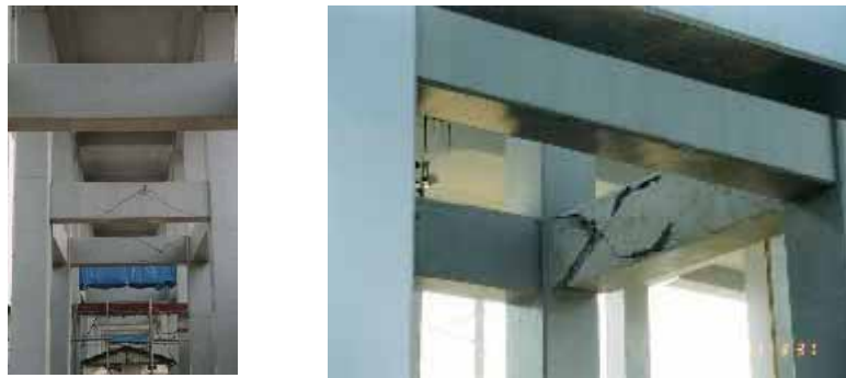
Photo.1 A damaged two story RC rigid frame elevated bridge of Sanyo Shinkansen
